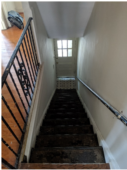
1 (Main Hall – View toward front entrance)
