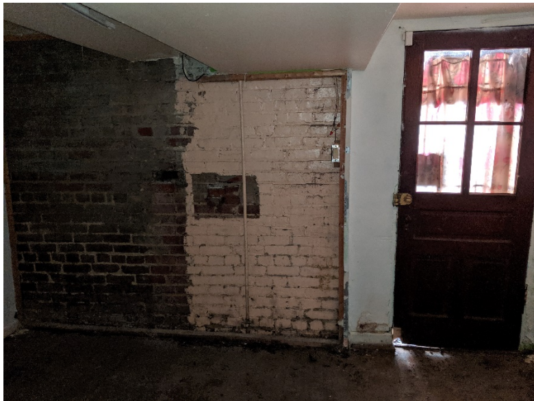
5 (View toward rear entrance)
