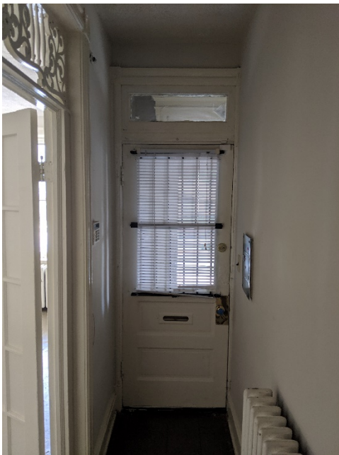
1 (Main Hall – View toward front entrance)
