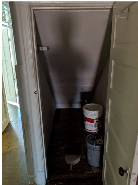
3 (Main Hall – View toward front entrance)
