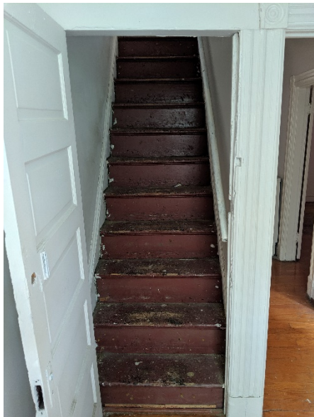
6 (View toward stair to third floor)
